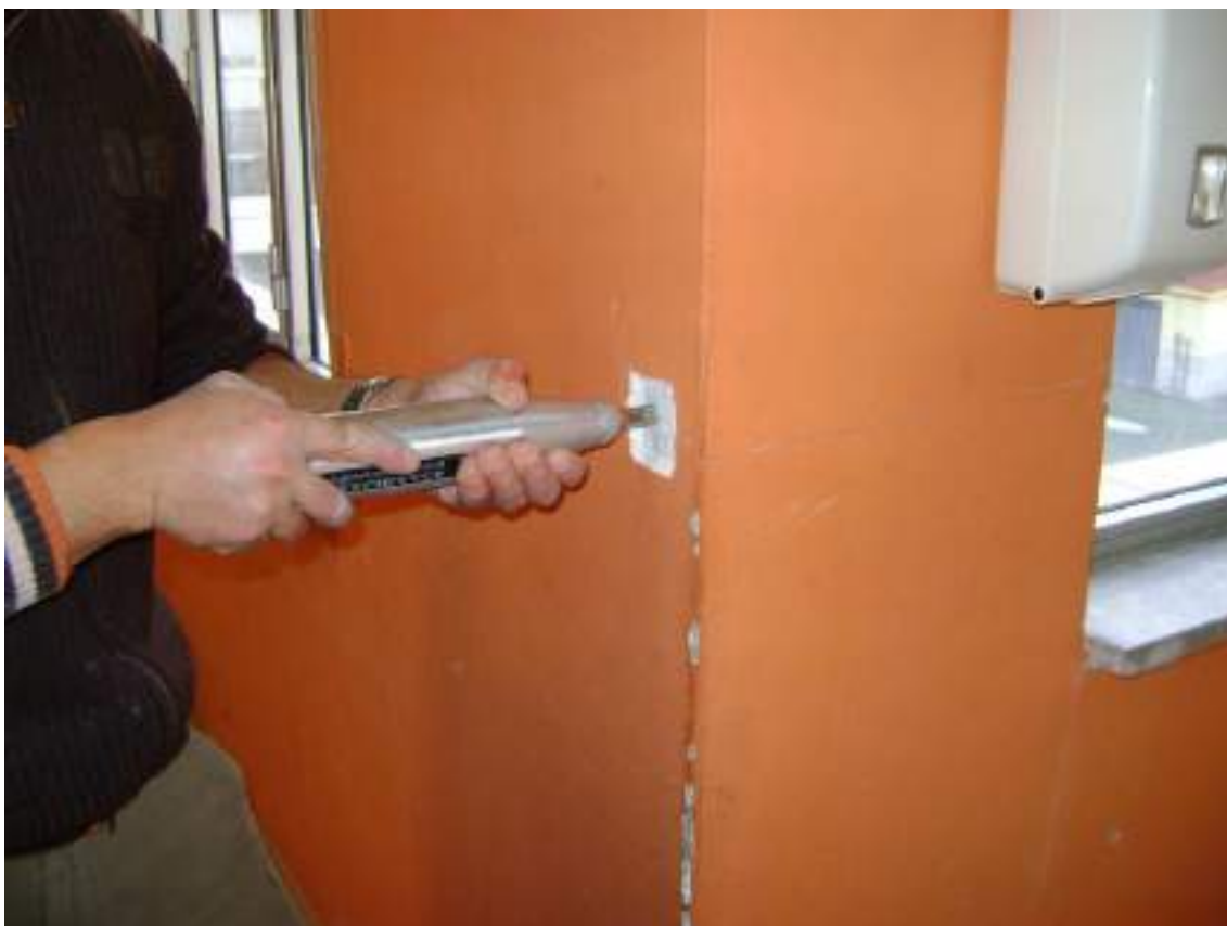
Figura 76 - Sclerometria pilastro P/1P/14
