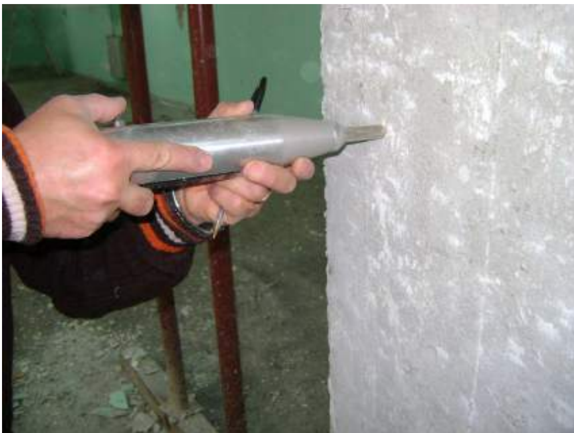
Figura 46 - Sclerometria pilastro P/PS/10
