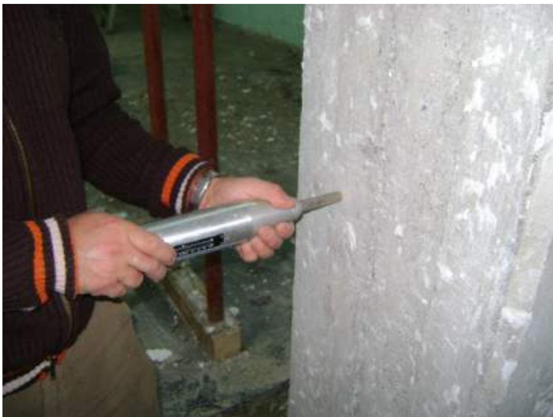
Figura 48 - Sclerometria pilastro P/PS/9
