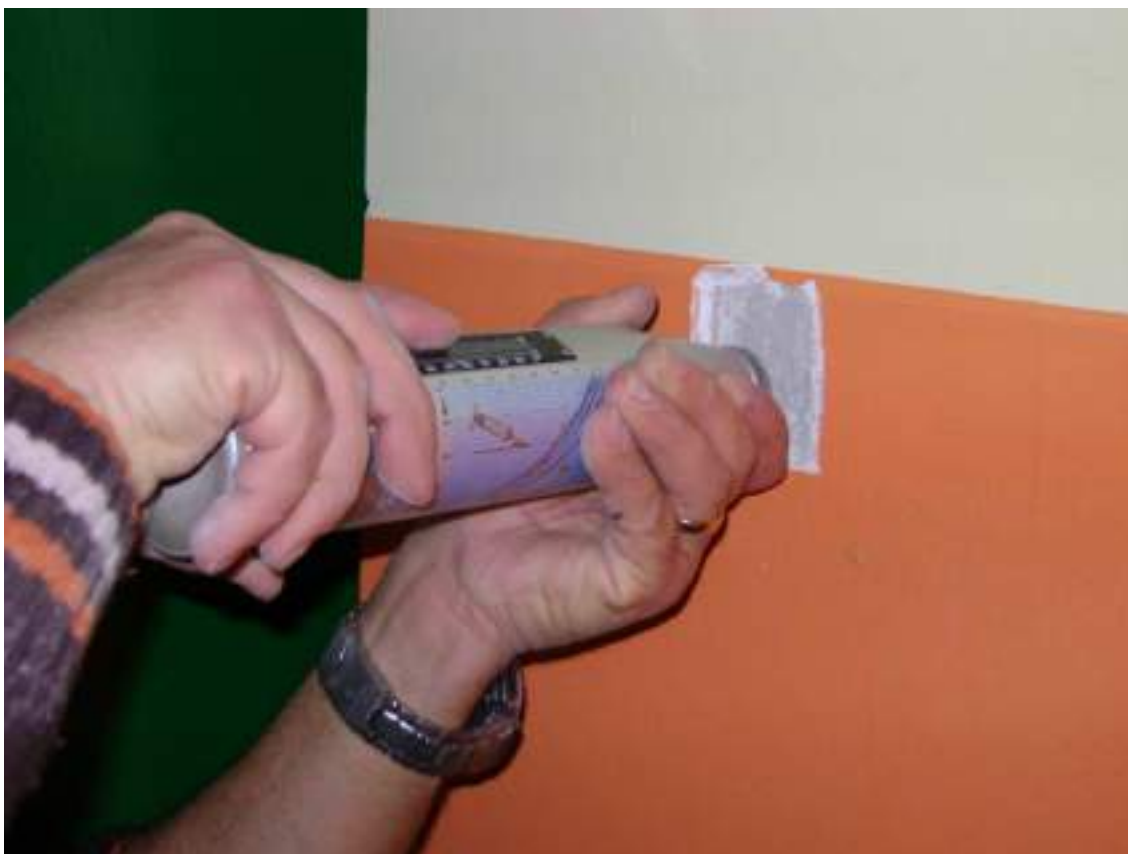
Figura 80 - Sclerometria pilastro P/1P/23
