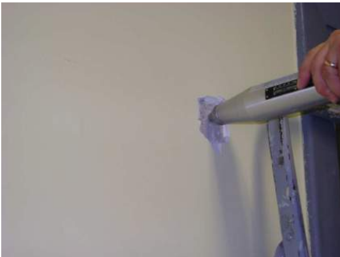
Figura 72 – Sclerometria pilastro P/1P/8
