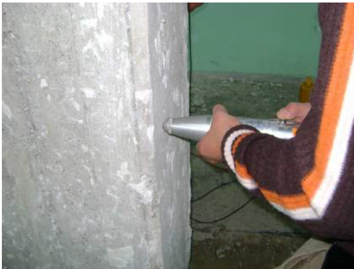
Figura 44 - Sclerometria pilastro P/PS/11
