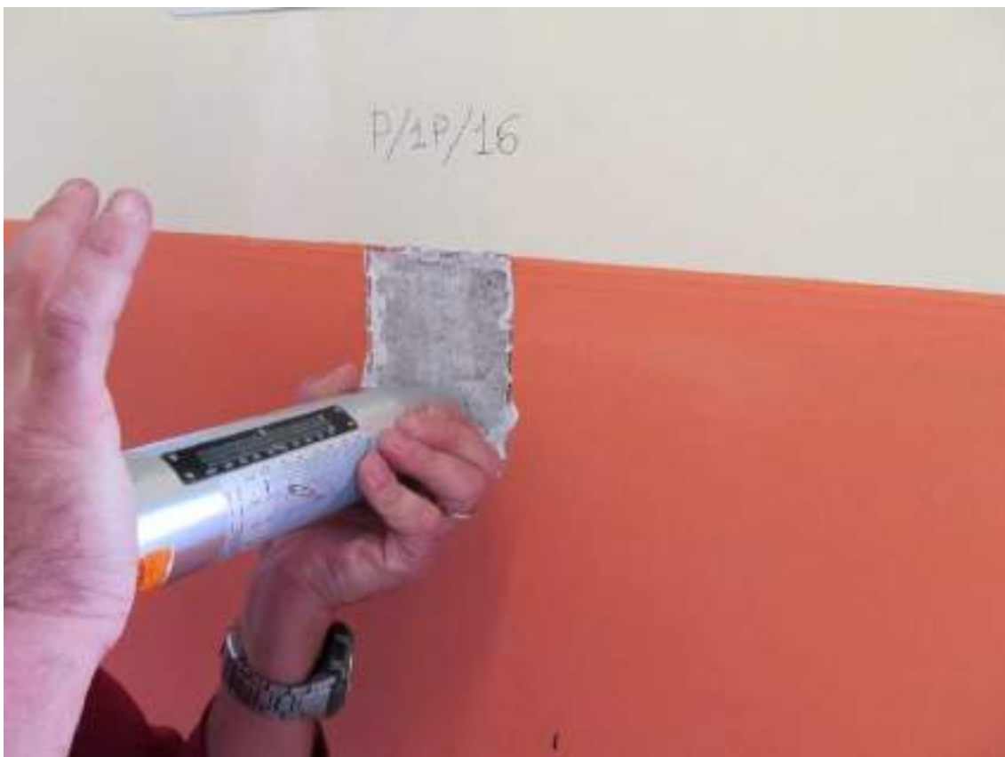
Figura 82 - Sclerometria pilastro P/1P/16
