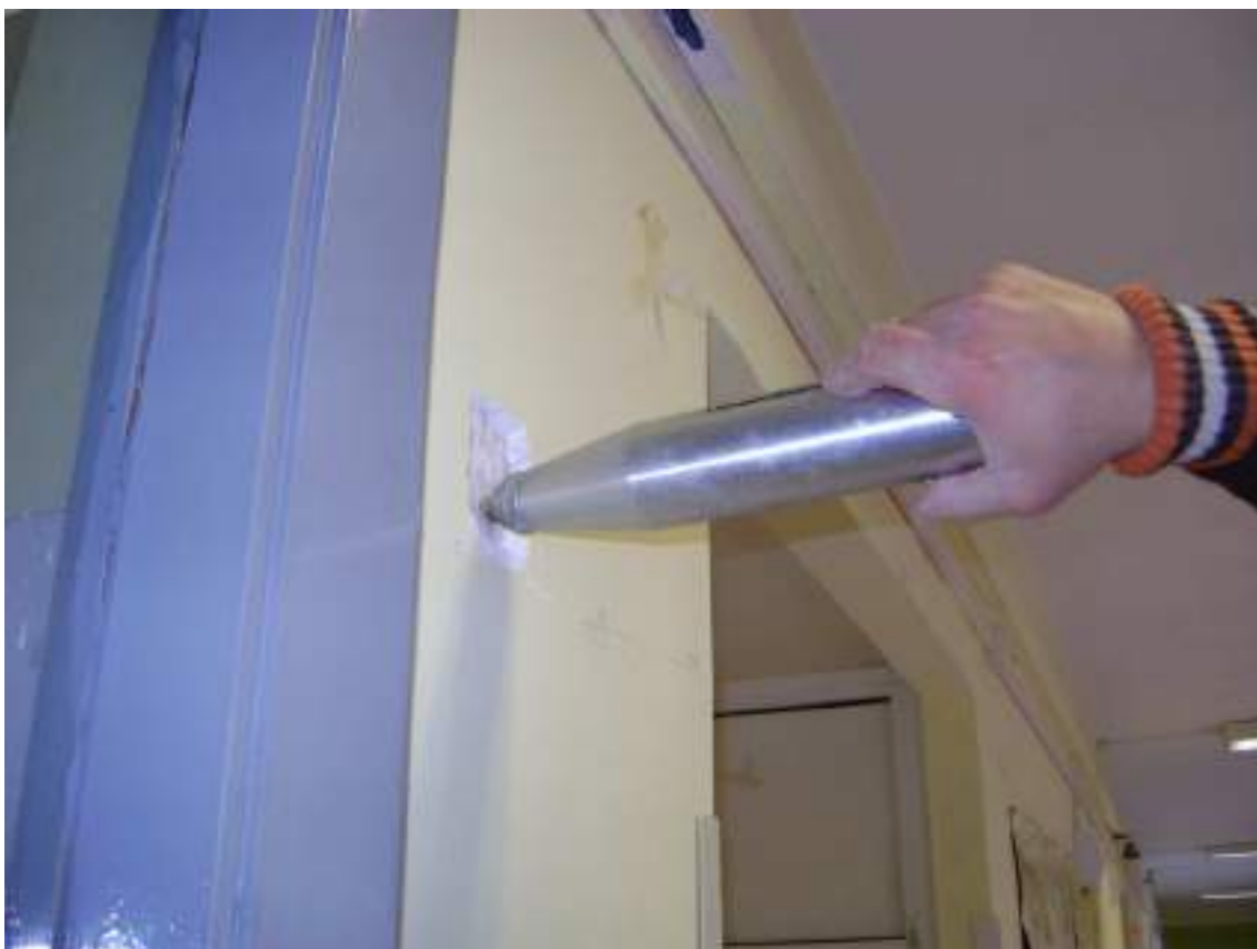
Figura 74 - Sclerometria pilastro P/1P/11
